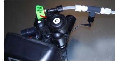
... PIPE INLET RESTORATION-BRINE
